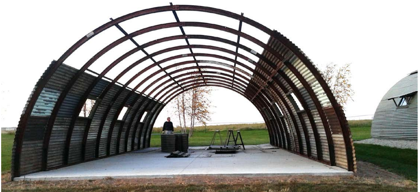
2nd WW II Quonset Hut under restoration and construction at Camp Hastings Military Museum, MN. by WW II HRS members and others. Photos Submitted by David Halseth 117th IR, 30th Div. USA
