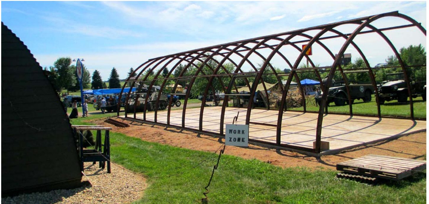
2nd WW II Quonset Hut under restoration and construction at Camp Hastings Military Museum, MN. by WW II HRS members and others. Photos Submitted by David Halseth 117th IR, 30th Div. USA
